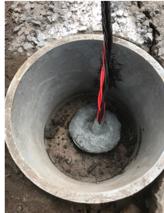
Photo of sand pocket before the sand and cold mix is added. Notice the pavement cut near the top of the picture where the wires come in from the roadway.
