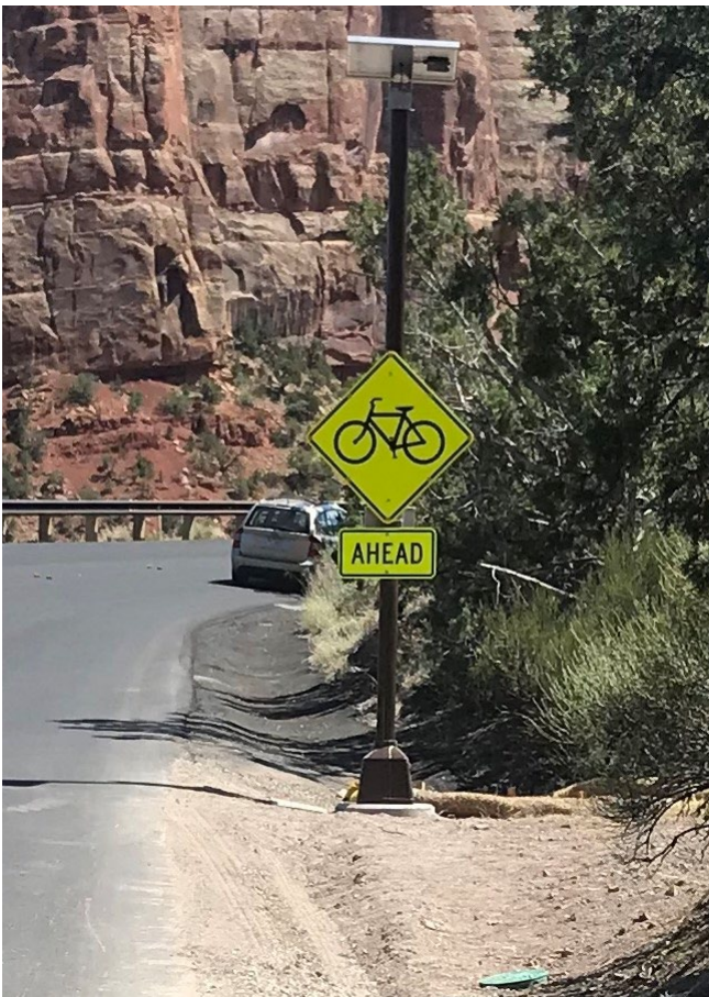
Figure 1: Colorado National Monument warning sign 1 with bicycle blinker panel (photo: WTI)
