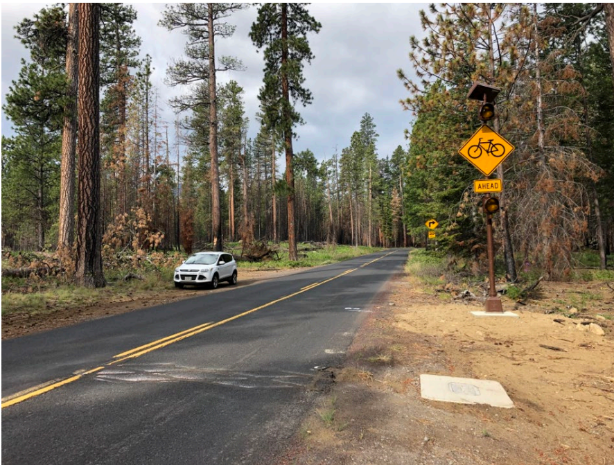
Figure 2: Hwy 242 warning sign near Milepost 84 with dual amber beacons near Sisters, Oregon (photo: WTI)
