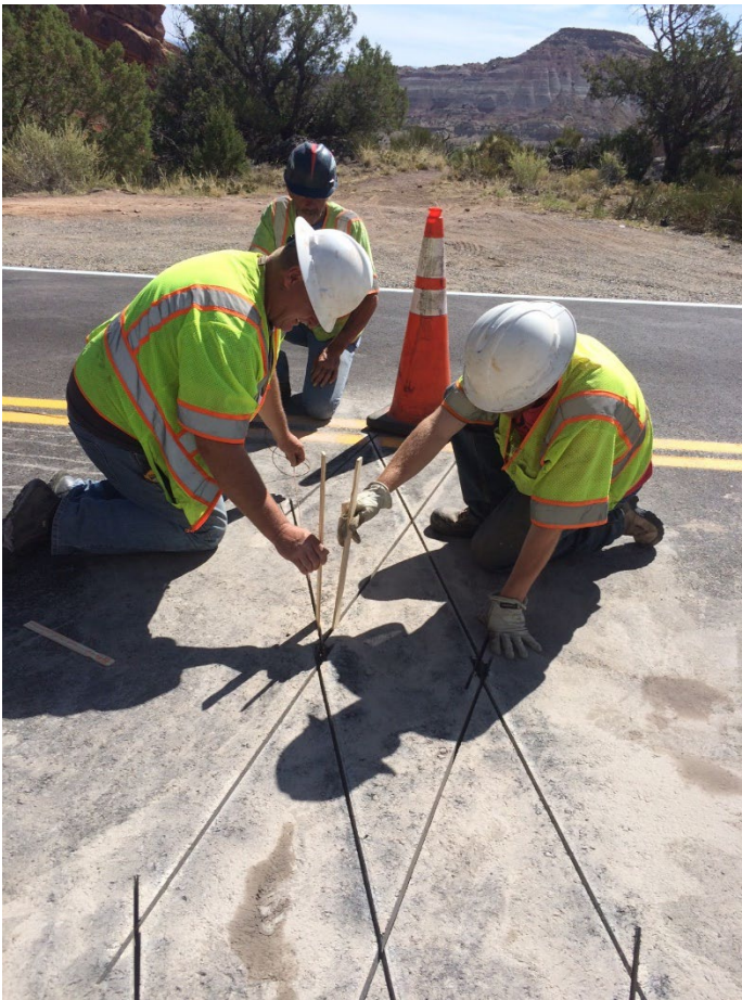
Figure 4: Contractor installing inductive loops for bicycle detection at Colorado National Monument (photo: WTI)
