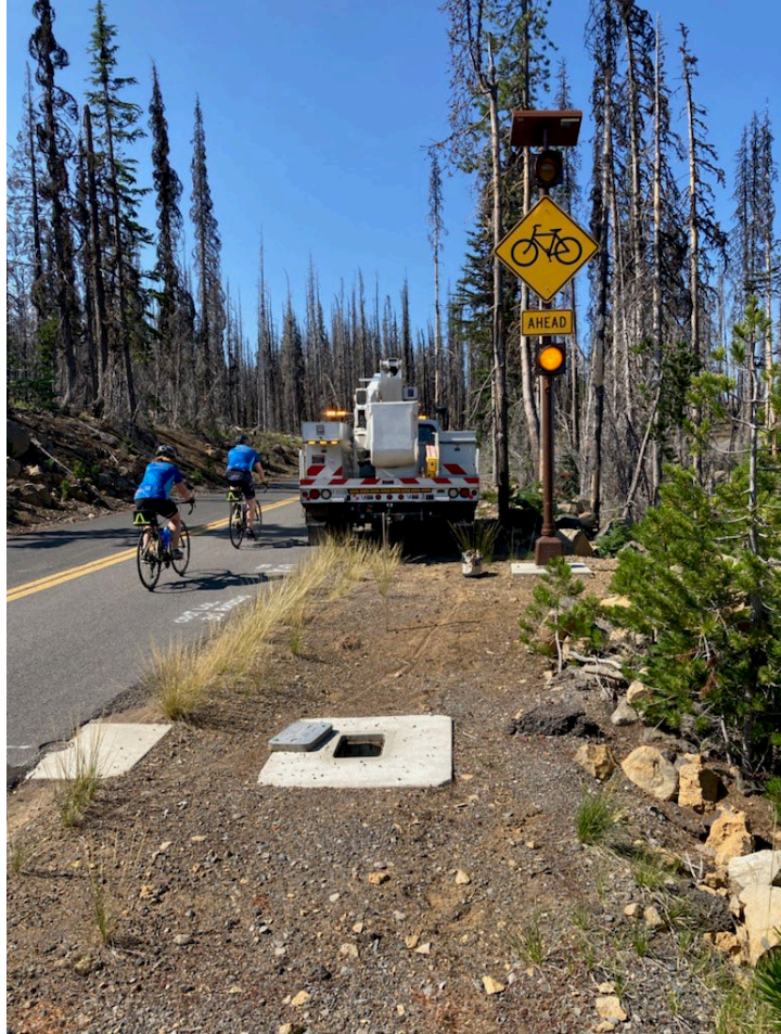
Figure 6: Oregon HWY 242 dynamic warning sign near Milepost 78 and concrete junction box (photo: ODOT)
