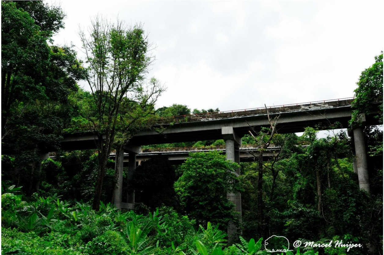
Figure 128. Tall bridges allow for light and moisture under the structure, and for continuous habitat for nearly all species, including small animal species, China.
