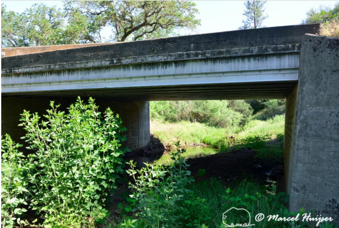
Figure 100. Bottomless multifunctional underpass, Hwy 88 near Jackson, California, USA. The underpass is for a creek (hydrology) and wildlife (e.g. mule deer).
