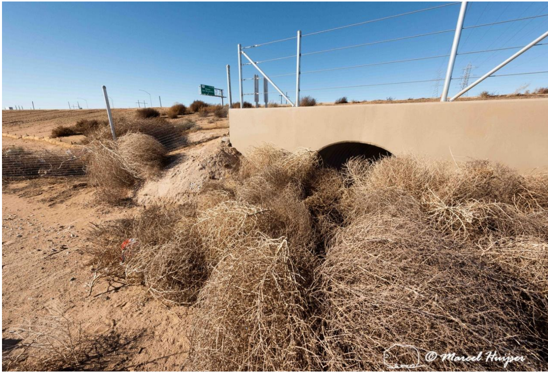
Figure 136. Tumbleweed blocks culverts, primarily for hydrology, but also for Mojave desert tortoise ( Gopherus agassizii ), Hwy 58 near Kramer Jct, California, USA.
