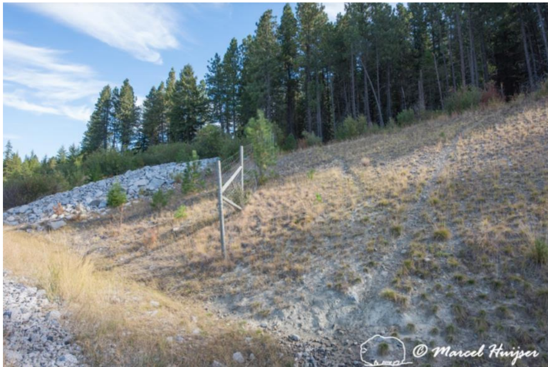
Figure 85. Wildlife trail at a fence-end, US Hwy 95, Bonners Ferry, Idaho, USA. This is an indication that there is a concentration of wildlife crossings at the fence-end (a “fence-end run”), potentially resulting in a concentration of collisions at or near the fence-end, just inside or just outside the fenced road section.
