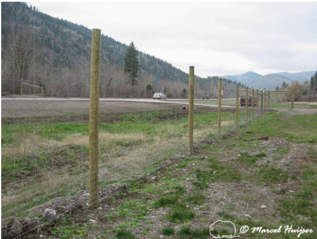
Figure 79. Typical large ungulate fence in North America, 8 ft tall, wooden posts and mesh-wire fence material, US Hwy 93 North, Montana, USA. Note that there is a dig barrier attached to the main fence material (e.g., for canids).
