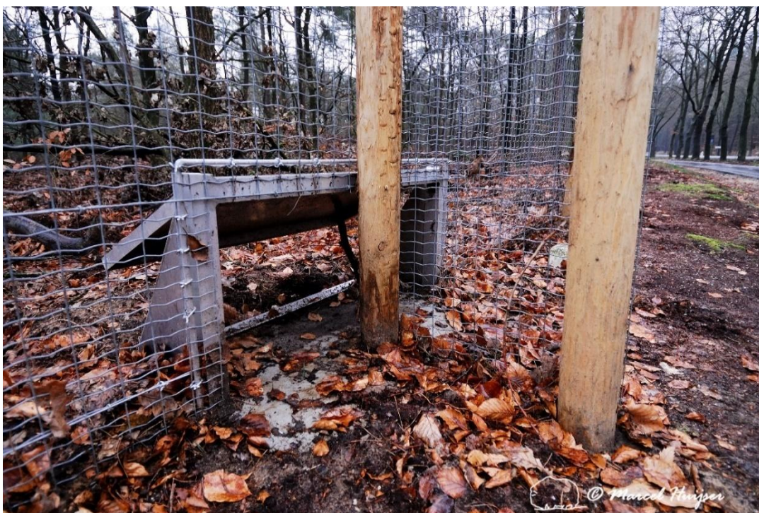
Figure 148. Escape gate for Eurasian badger ( Meles meles ) in wildlife fence Harderwijk, The Netherlands. Note that these types of gates are often left open because of debris which threatens their functioning.
