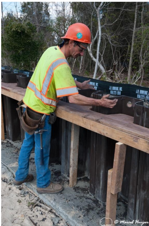
Figure 106. Barrier wall for turtles, alligators, snakes and amphibians, Lake Jackson Ecopassage, Tallahassee, Florida, USA. The barrier wall was under construction when the image was made.
