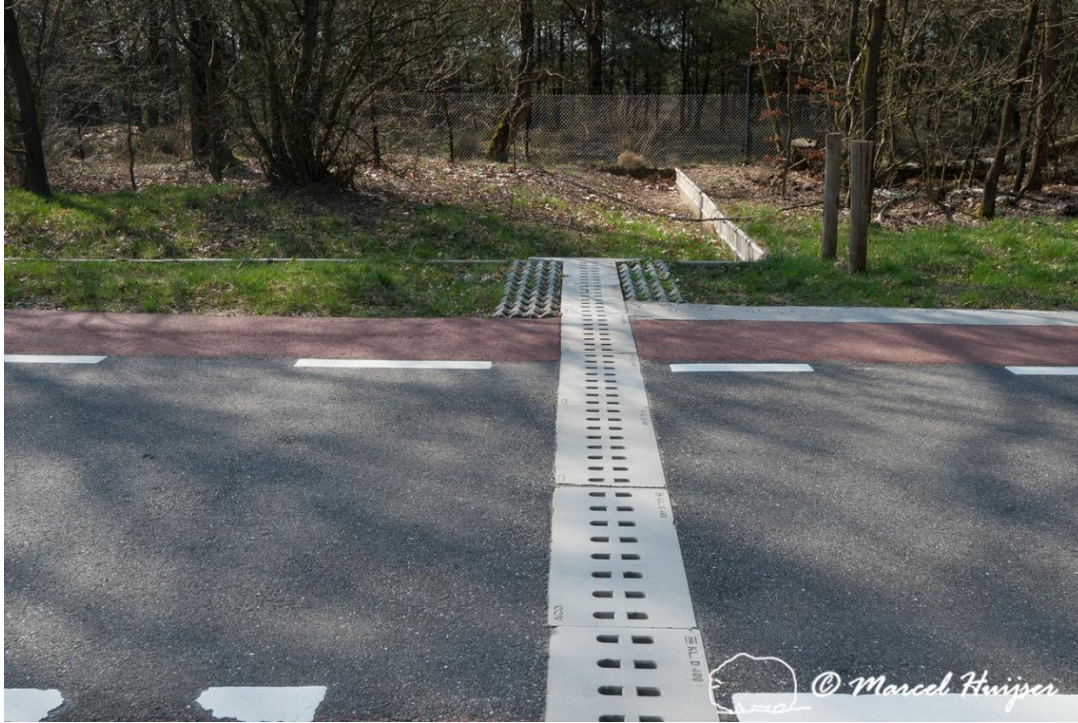
Figure 137. Amphibian tunnel with open slotted roof and barrier or wall for amphibians, integrated into roadbed, Deelenseweg, between Hoenderloo and Arnhem, Gelderland, The Netherlands.
