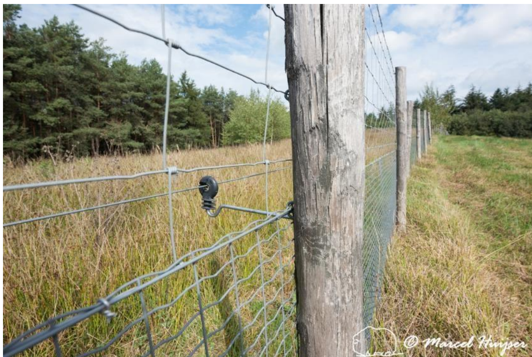
Figure 83: Wildlife fence along A28 motorway, near Spier, Drenthe, The Netherlands. The fence is a barrier for medium and large mammal species. The electrified wire is an additional barrier to keep animals out of the fenced road corridor.
