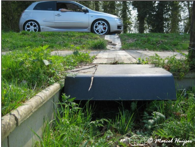
Figure 129. Cover close to the entrance of an amphibian tunnel, The Netherlands.
