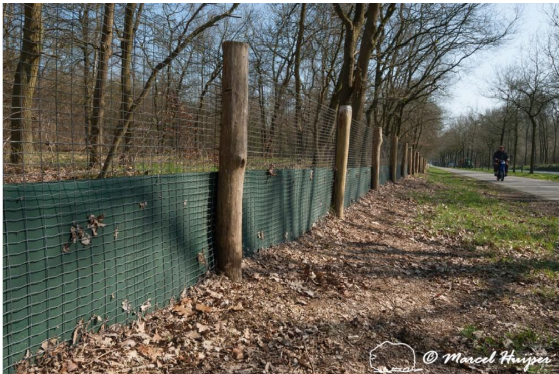
Figure 102. A “fence” designed for Eurasian badger ( Meles meles ) (the taller metal fence material with small mesh size) and for common toad ( Bufo bufo ) (the plastic sheets at the bottom of the fence), Rijksweg Elsterstraatweg N225 just west of Elst, Utrecht, The Netherlands.
