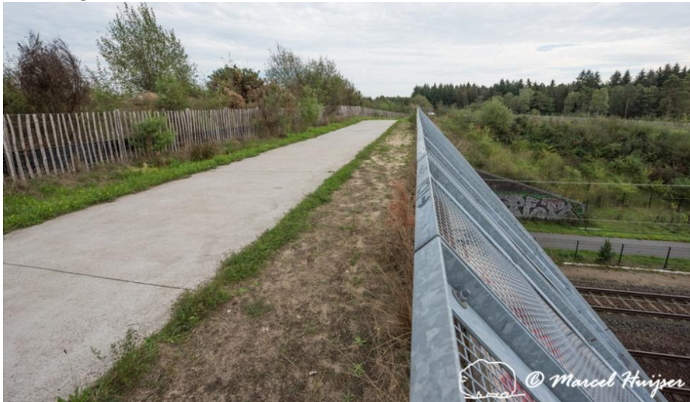
Figure 98. Hiking and biking trail combined with wildlife overpass across railroad tracks, Soest, The Netherlands. The “wildlife area” on the overpass is further to the left, separated from the trail by a berm and shrubs and trees.
