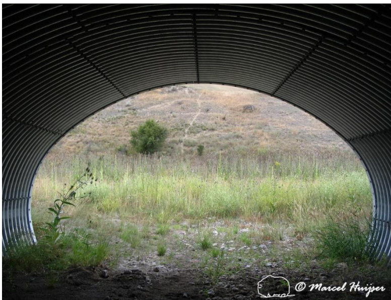
Figure 123. Corrugated metal culvert with bottom placed below the ground level of the surroundings, US Hwy 93, near Ravalli, Flathead Indian Reservation, Montana, USA.
