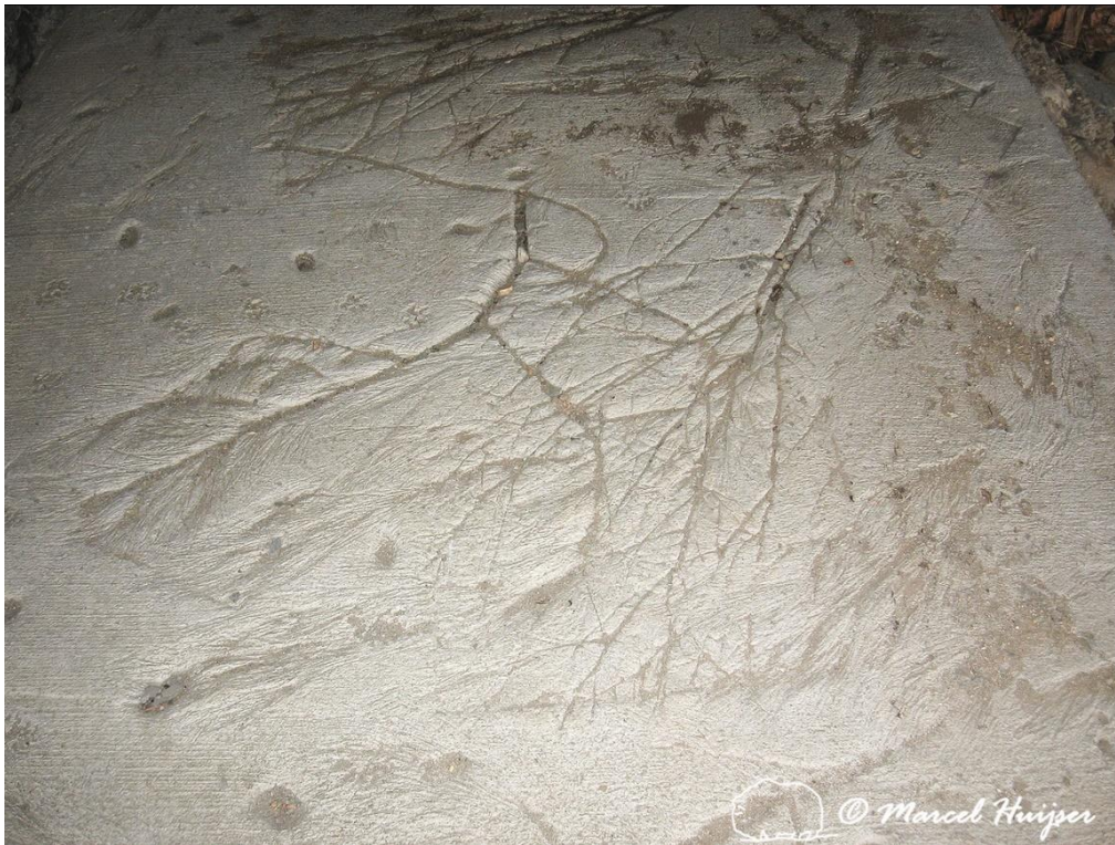
Figure 135. Imprints in concrete surface in wildlife underpass to make it less slippery for wildlife, US Hwy 93 S, Bitterroot Valley, Montana, USA.
