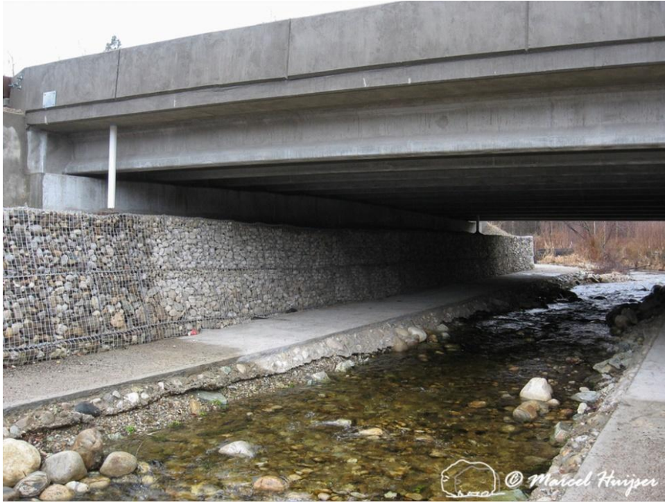
Figure 99. Pathway for large mammals in an underpass (bridge) primarily designed for water (stream), US Hwy 93 S, Bitterroot Valley, Montana, USA.
