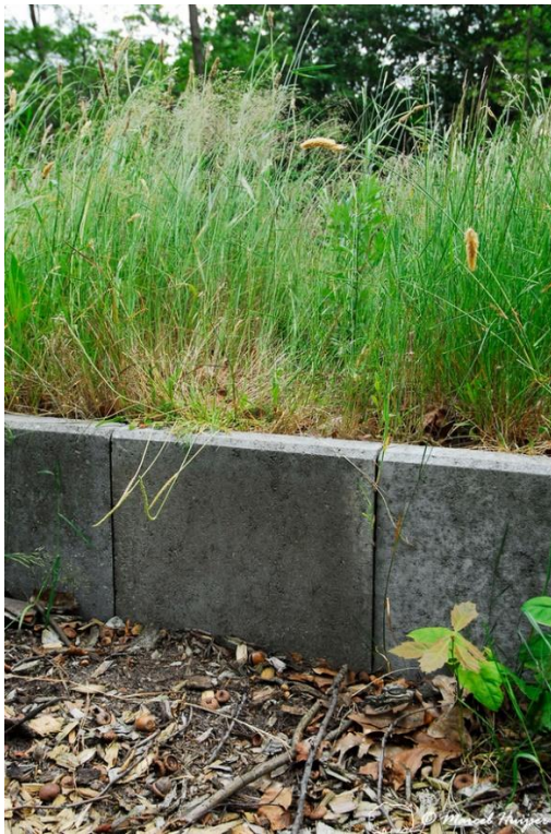
Figure 107. A “barrier wall” (concrete) integrated into the roadbed for common toads ( Bufo bufo ), Deelenseweg, between Hoenderloo and Arnhem, Gelderland, The Netherlands.
