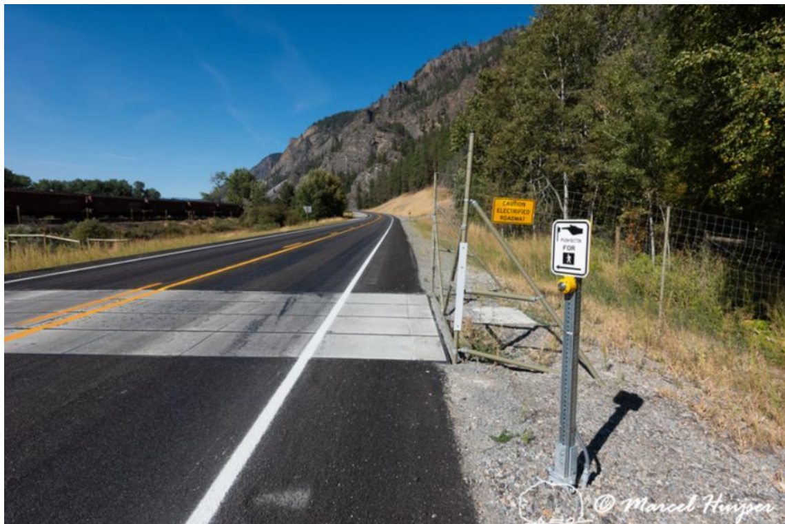
Figure 87. Electrified barrier embedded in travel lanes to keep large mammals, including bighorn sheep, out of fenced road corridor, MT Hwy 200, Thompson Falls, Montana, USA.
