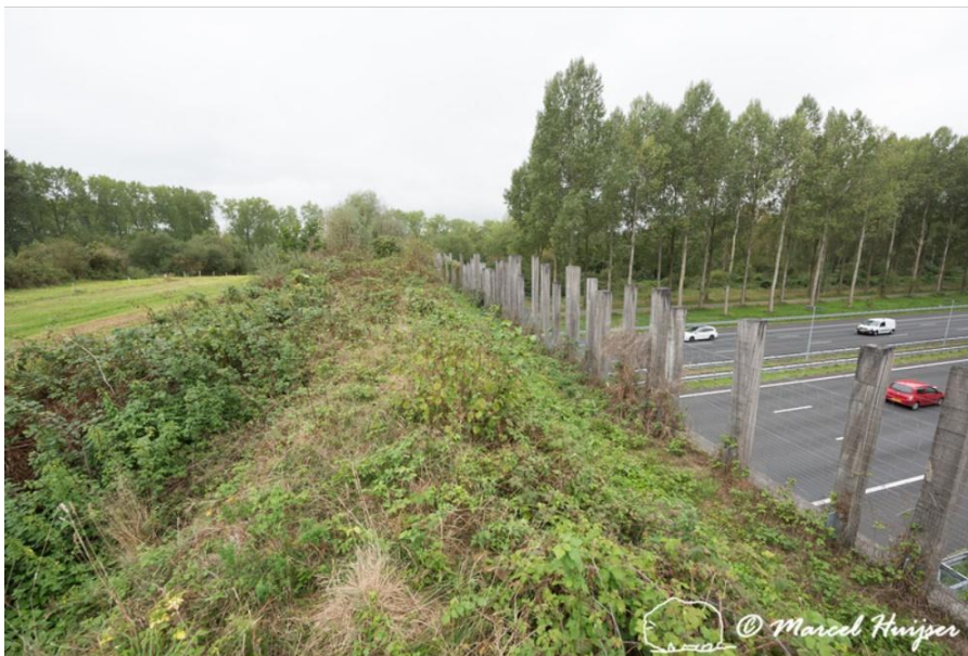
Figure 94. Berm on wildlife overpass "Groene Woud" across A2 motorway, The Netherlands. The berm with rootwads and shrubs provides cover on either side and reduces visual and noise disturbance barrier combined with large mammal fence on an overpass, The Netherlands.
