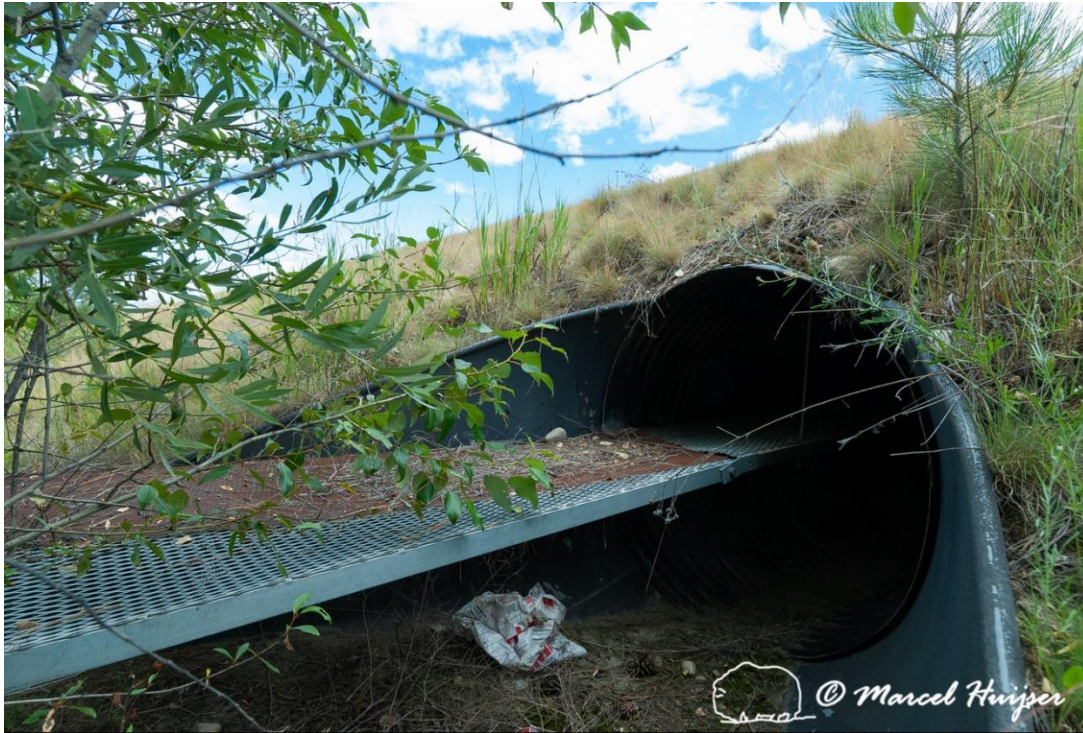
Figure 134. Shelf for small mammals in culvert originally designed for hydrology only, US Hwy 93 South, Montana, USA.
