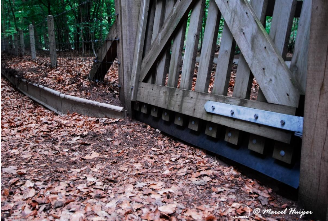
Figure 144. A gate for pedestrians and bicyclists at a barrier wall for amphibians, The Netherlands. The rubber flap is designed to keep common toads ( Bufo bufo ) from crawling under the gate and gaining access to the main road.
