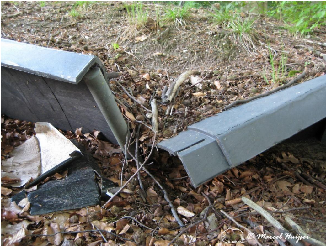
Figure 150. A barrier wall for common toads ( Bufo bufo ) has collapsed, The Netherlands.
