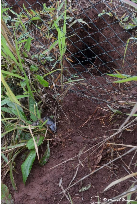
Figure 151. An animal (probably a nine-banded armadillo ( Dasypus novemcinctus )) dug a gap under a wildlife fence. The burrow is visible on roadside of the fence, SP-225 motorway, near Brotas, São Paulo, Brazil.
