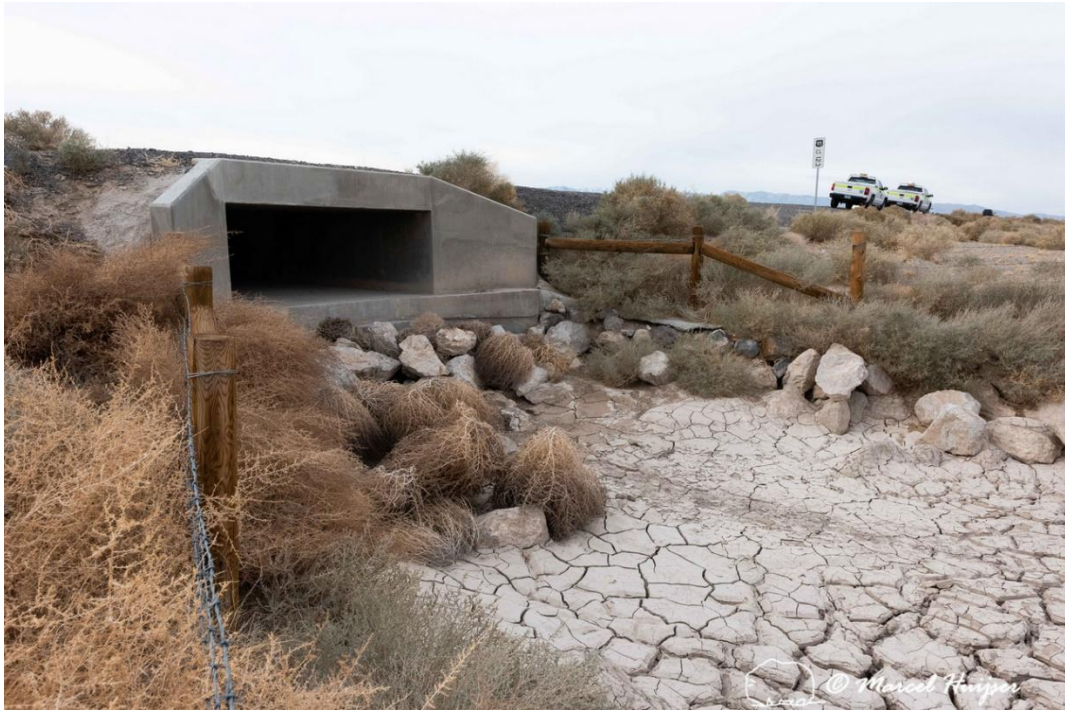
Figure 153. A culvert with a heavily eroded outflow near Indian Springs, Nevada, USA. Inaccessible to desert tortoises.
