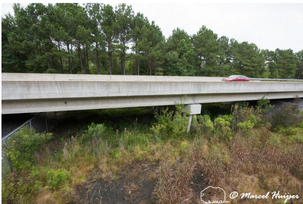
Figure 120. Wildlife underpass and fence with grasses, shrubs, and trees in the median and also some under the bridges, US Hwy 64, near Roper, North Carolina, USA.
