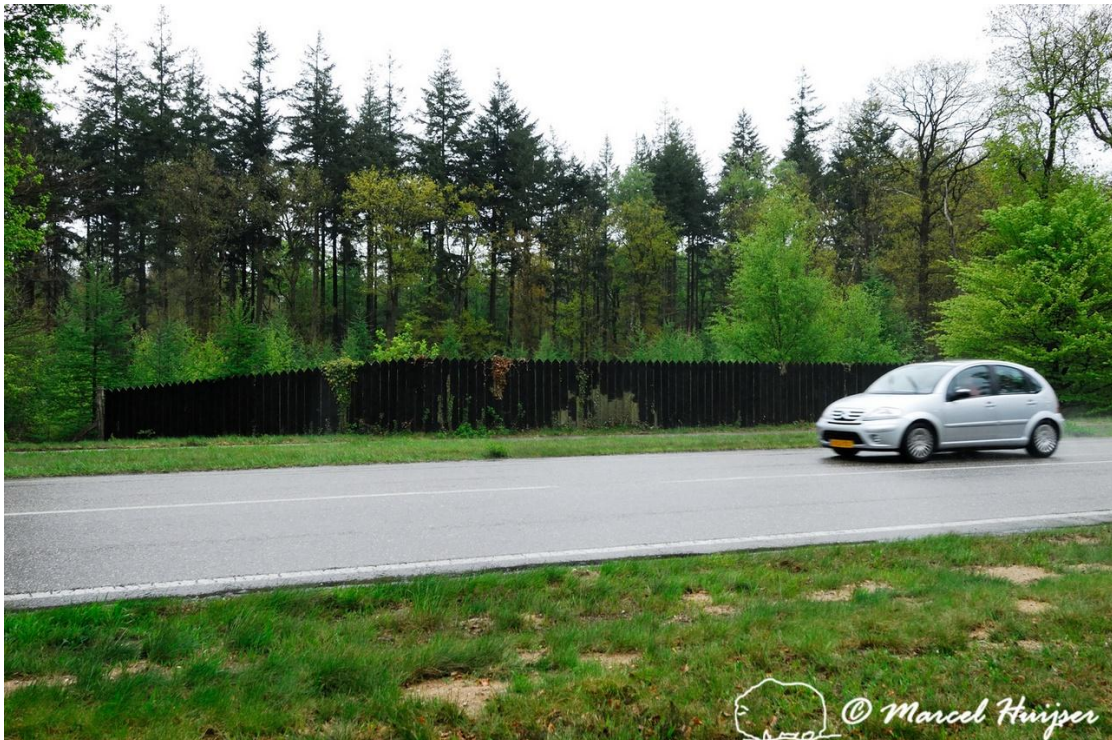
Figure 95. Visual barrier above a wildlife underpass, Amersfoortseweg, Hoog Soeren, The Netherlands. The fence reduces visual and noise disturbance from traffic for the animals that approach the underpass.
