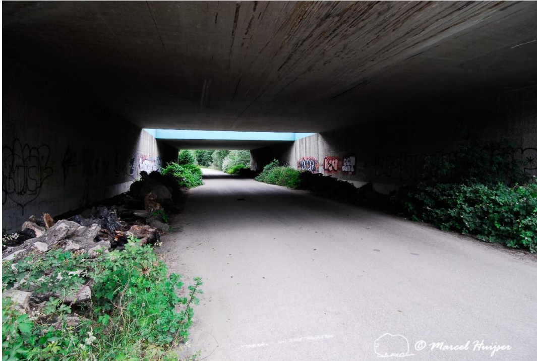
Figure 140. An existing underpass for a low volume road under a 4-lane A27 motorway, near Hilversum, The Netherlands. The structure was made more suitable for small animal species by placing rows of root wads along the sides.
