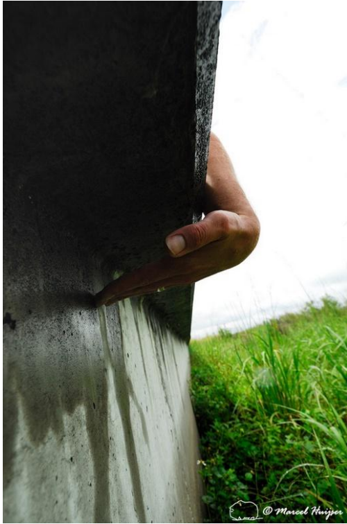
Figure 113. Barrier wall integrated into the roadbed with overhang for reptiles, amphibians and small mammals, U.S. 441, Paynes Prairie Ecopassage, south of Gainesville, Florida, USA.
