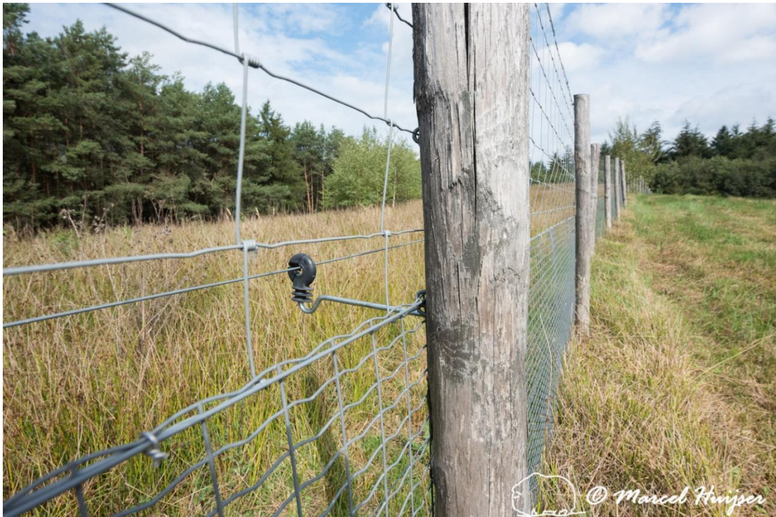
Figure 117. Wildlife fence along A28 motorway, near Spier, Drenthe, The Netherlands. The fence is a barrier for medium and large mammal species. The electrified wire is an additional barrier to keep animals from climbing the fence.
