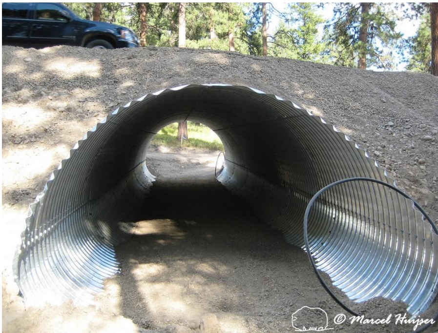
Figure 121. Corrugated metal culvert with soil covering the bottom.
