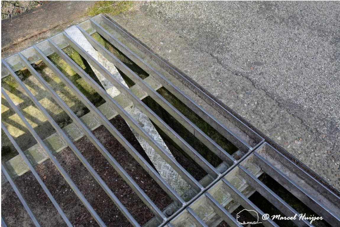
Figure 146. Escape ramp for small animals from pit under wildlife guard National Park Hoge Veluwe, The Netherlands.
