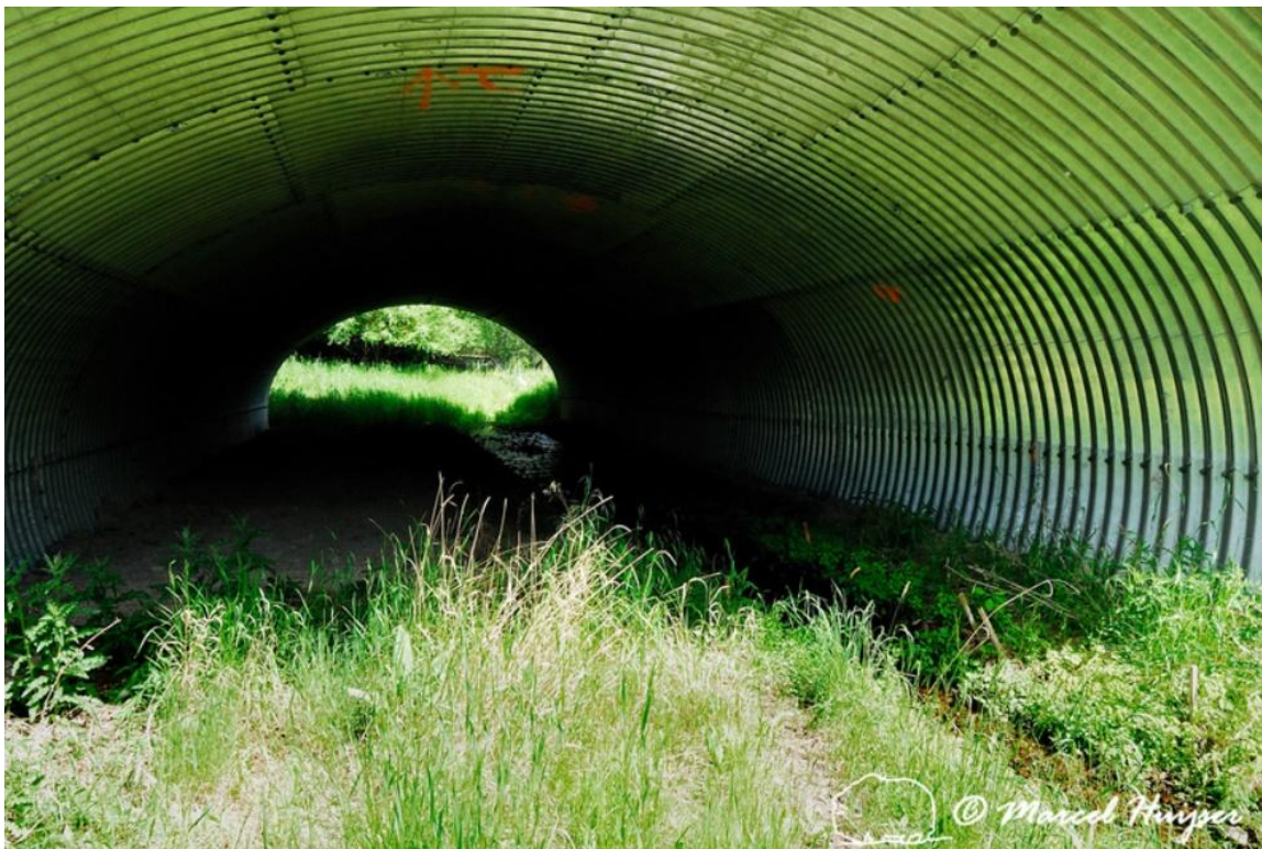
Figure 101. Multi-functional underpass for wildlife and water with soil and rocks that cover the bottom of the culvert, US Hwy 93, near St Ignatius, Flathead Indian Reservation, Montana, USA.
