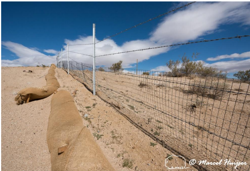
Figure 108. Fence to keep desert tortoise ( Gopherus agassizii ) off the highway, California, USA.
