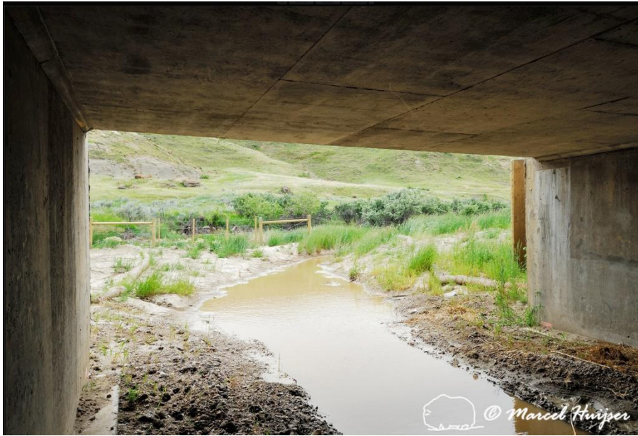
Figure 122. Bottomless culvert.
