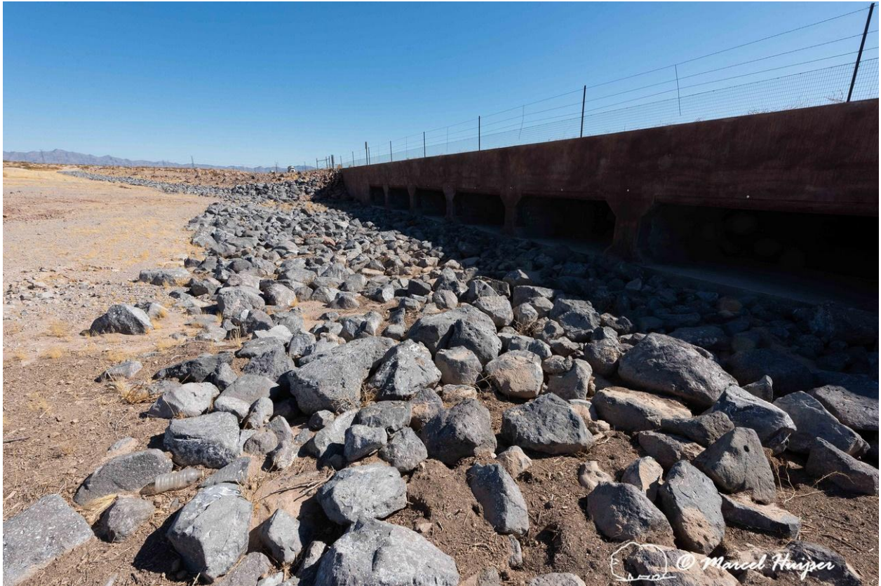
Figure 149. Riprap in front of culverts to reduce erosion, but the boulder are a barrier to Mojave desert tortoise ( Gopherus agassizii ), I-11, near Boulder City, Nevada, USA.
