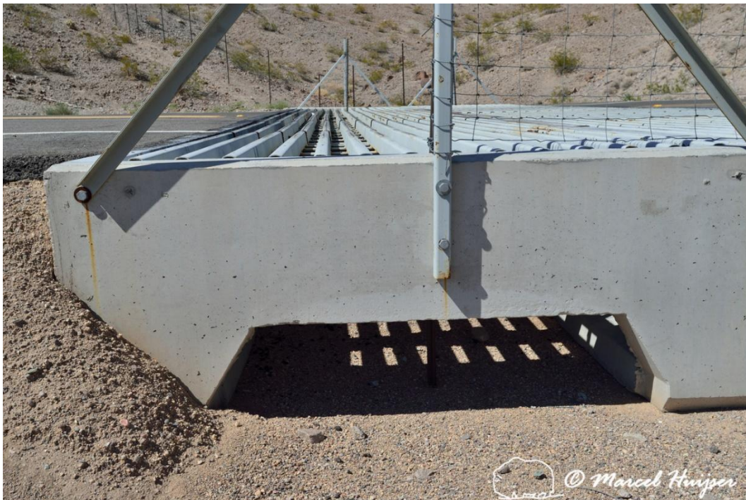
Figure 145. Combined drainage and escape for small animals under wildlife guard, Arizona, USA. The openings on the side allow for drainage under the culvert. The openings also allow invertebrates, amphibians, reptiles, small mammals and other species that may fall in between the metal bars to escape. For wildlife guards that have a fully enclosed pit with contiguous walls sometimes wooden planks or metal strips are attached, allowing animals to climb out of the pit.
