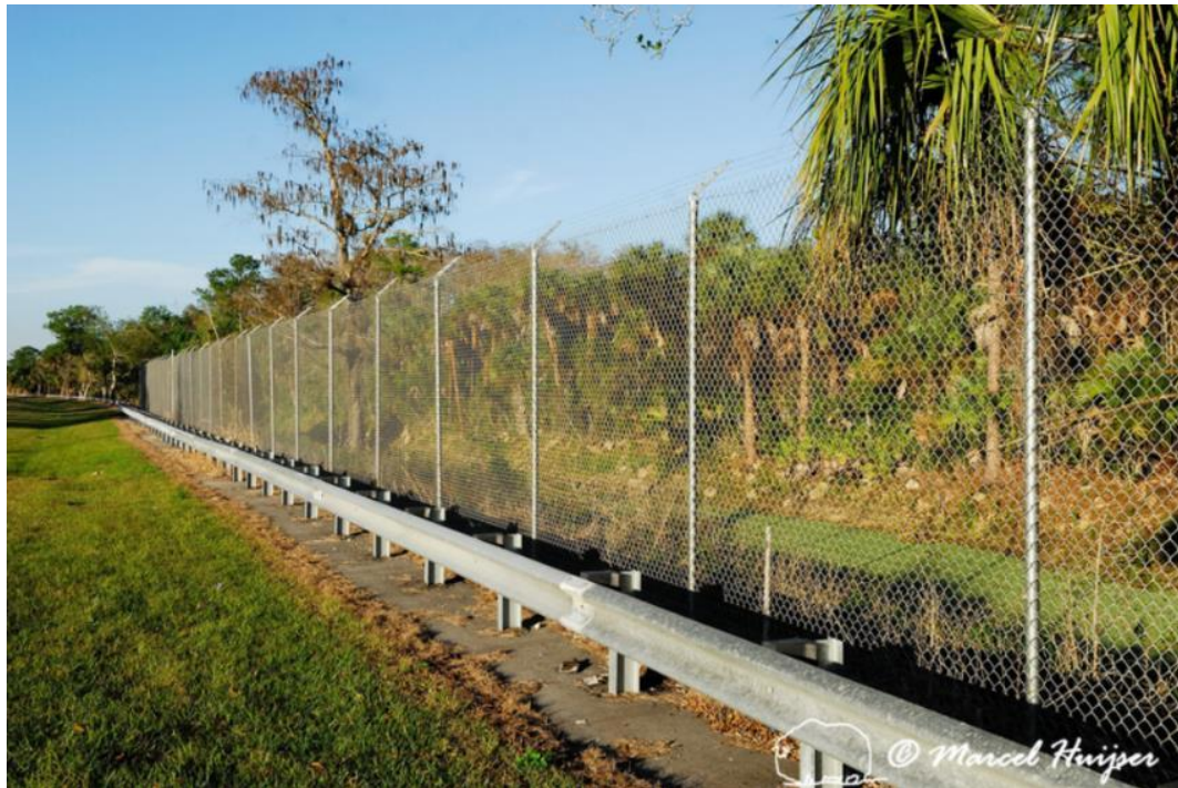
Figure 80. Fence for Florida panther ( Puma concolor coryi ), 10 ft tall, metal posts, chain-link fence material, and overhang or outrigger, SR 29, Florida, USA).
