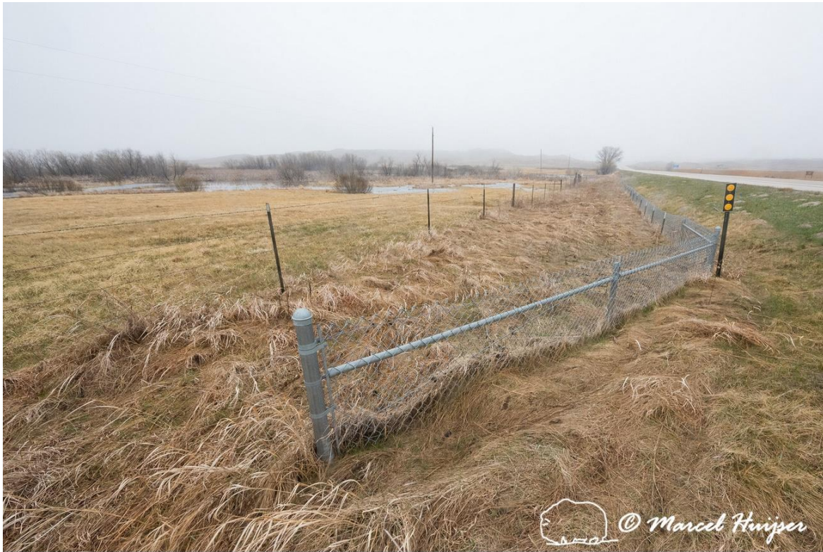
Figure 143. Though not meeting the recommended specifications for a “turn-around fence-end”, this is an attempt at discouraging turtles from crossing the road in high numbers at the fence-end, US Hwy 83, Valentine National Wildlife Refuge, Nebraska, USA.
