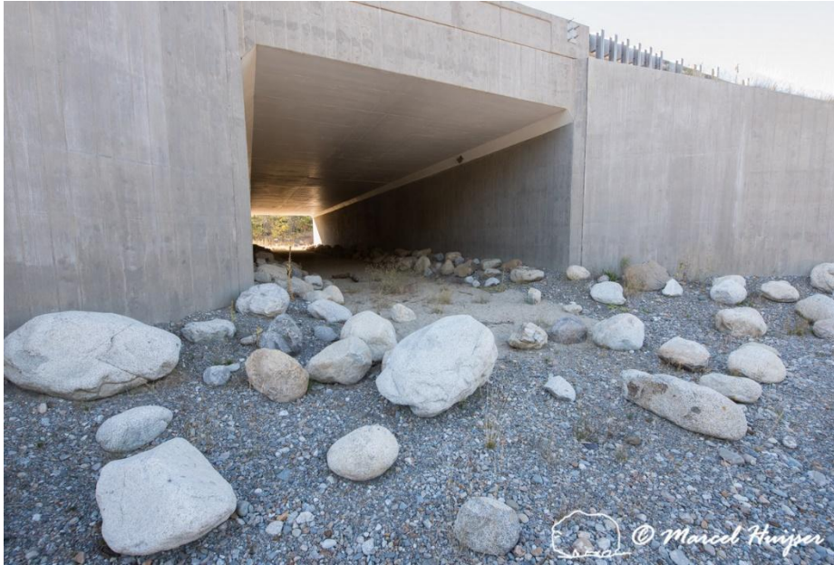
Figure 132. Boulders provide cover to small animal species and block access to unauthorized vehicles at wildlife underpass, US Hwy 95, Chilco, Idaho, USA.
